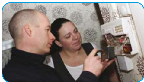
Installing new monitored alarms
