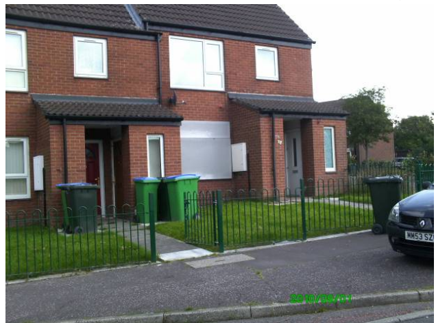
The Cray flats after new fencing
