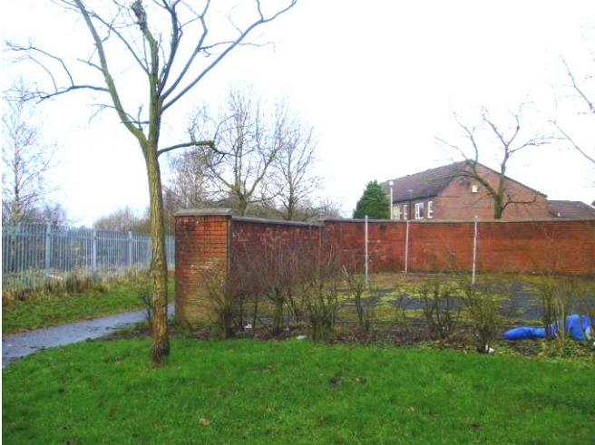
Laythe Barn drying area with brick wall
